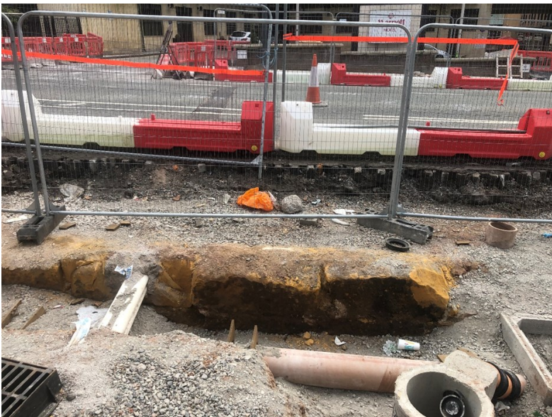
Wall exposed during the excavation of a drainage trench
