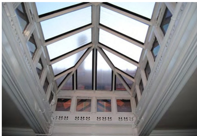
Glazed lantern above the central hall within Mossley House (©Turley Heritage)
