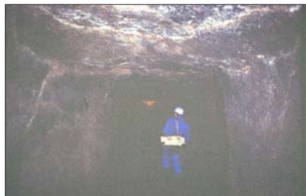
Change in tunnel dimensions from wide width to narrower passageway
