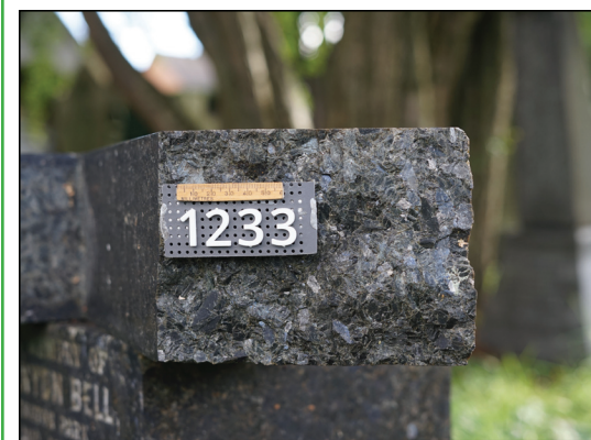
A broken larvikite cross shaft
