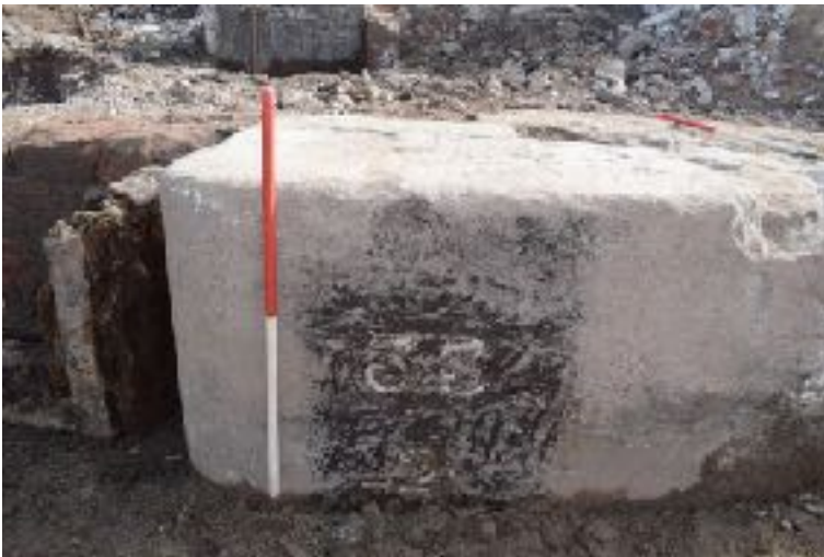
Figure 5. Depth gauge carved into the entrance lock wall and indicating a depth of 32 feet to the base of the lock.
