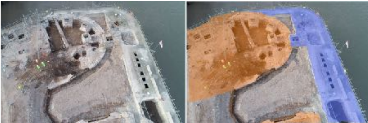
Figure 2. Overhead view of the excavation of Lyster's south lock-gate island showing the cross-walls and square shafts connected to the sluices. Two sets of gates were found in the infilled central lock, those on the left are closed, those on the right open. The image on the right has the 1860s works shaded orange, the 1949 works are shaded blue. The lock-gates are shaded brown.
