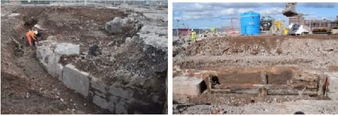
Figure 4. A Headland archaeologist cleaning one of the wooden lock-gates exposed after careful machine excavation and a lock-gate after cleaning.
