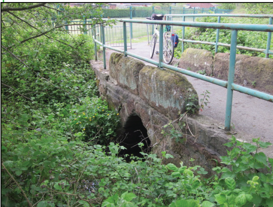
Two Butt Bridge Rainhill
