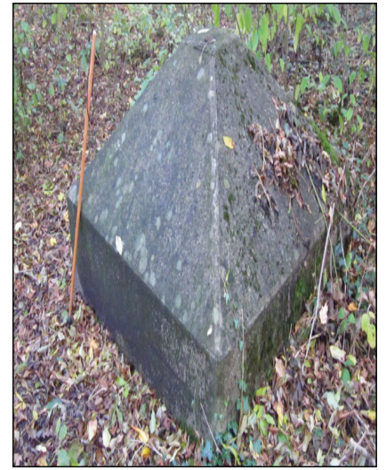
Capped Coal Mine Shaft - Alexandra Colliery
