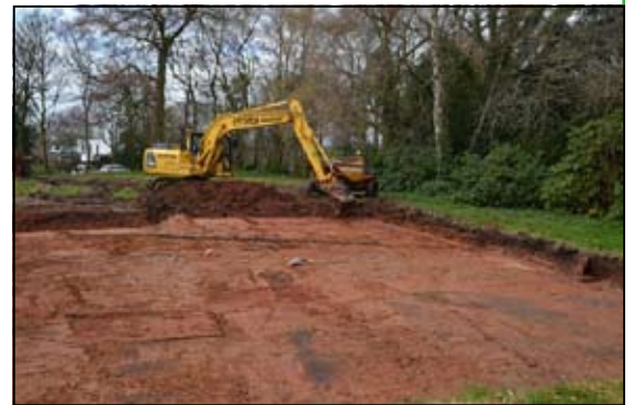
Top soil stripping in progress
