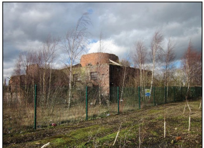
Cannington Shaw Bottle Shop, St Helens. A Scheduled Monument which is listed Grade II and is a building 'at risk'. It sits forlornly in a Tesco Car Park, neglected and ruinous. The St Helens Heritage Network has formed a group to obtain funding to adapt and reuse the building
