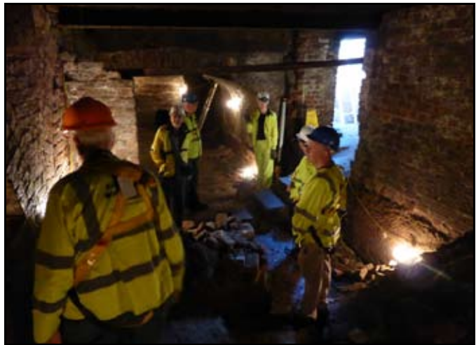
The 'Wine Bins' cellar below Williamson's House (photo I. Jones)
