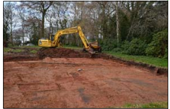
Top soil stripping in progress
