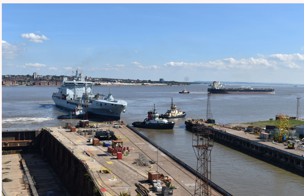
View of the Naval Ships entering the adjoining graving docks from the Priory tower
