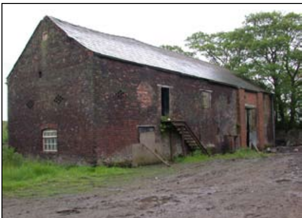
Fig. 2.30: Barn (Building 4) from north-west, May 2002
