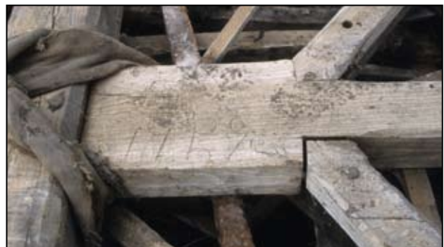
Fig. 2.31: Building 4, '1757' carved on roof timber, during demolition
