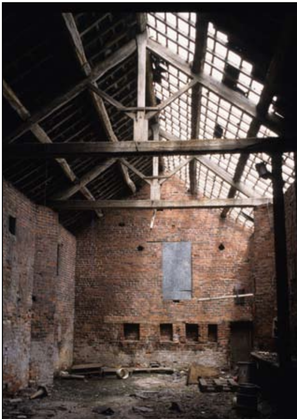
Fig. 2.33: Interior of barn (Building 4) after removal of slates
