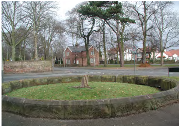
Figure 1. Modern view of the stone retaining wall which was constructed in 1845 to hold six of The Calderstones with Calder Cottage in the background.
