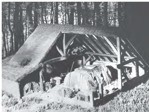
Fig. 6. Reconstruction of a wood-fired glasshouse based on the Blunden's Wood, Surrey c. 1330 excavation
